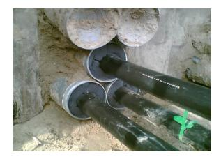
Duct sealing systems MD3 have been developed to an provide effective and simple solution for Gas and Watertight sealing of cables / pipes in ducts or bore holes.
